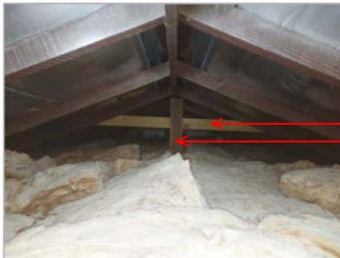
Photo 5. Extra strut under original ridge board
