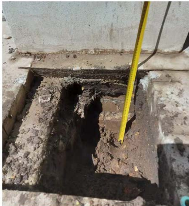
Photo 1. Exposed original brick footing in good condition
