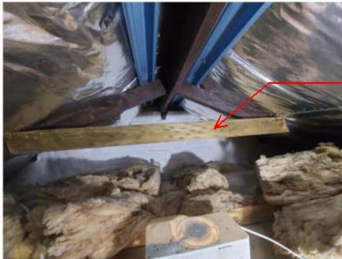
Photo 4. Extra pine collar ties fixed between original rafters
